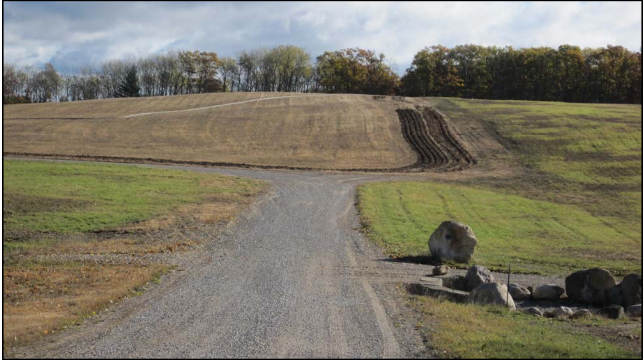
HOSE STRETCHED TO PLANNED INJECTION FIELD NOTE – SCARAFIED PERIMETER ON FIELD ABOVE
