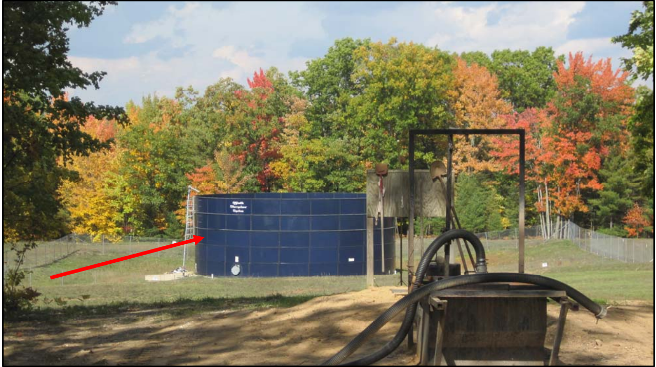
5-RING SLURRYSTORE (APPROXIMATELY 100,000-GALLONS/RING) THIS SLURRYSTORE HAS THE ABILITY OF 2-ADDITIONAL RINGS (OVER 700,000-GALLONS)
