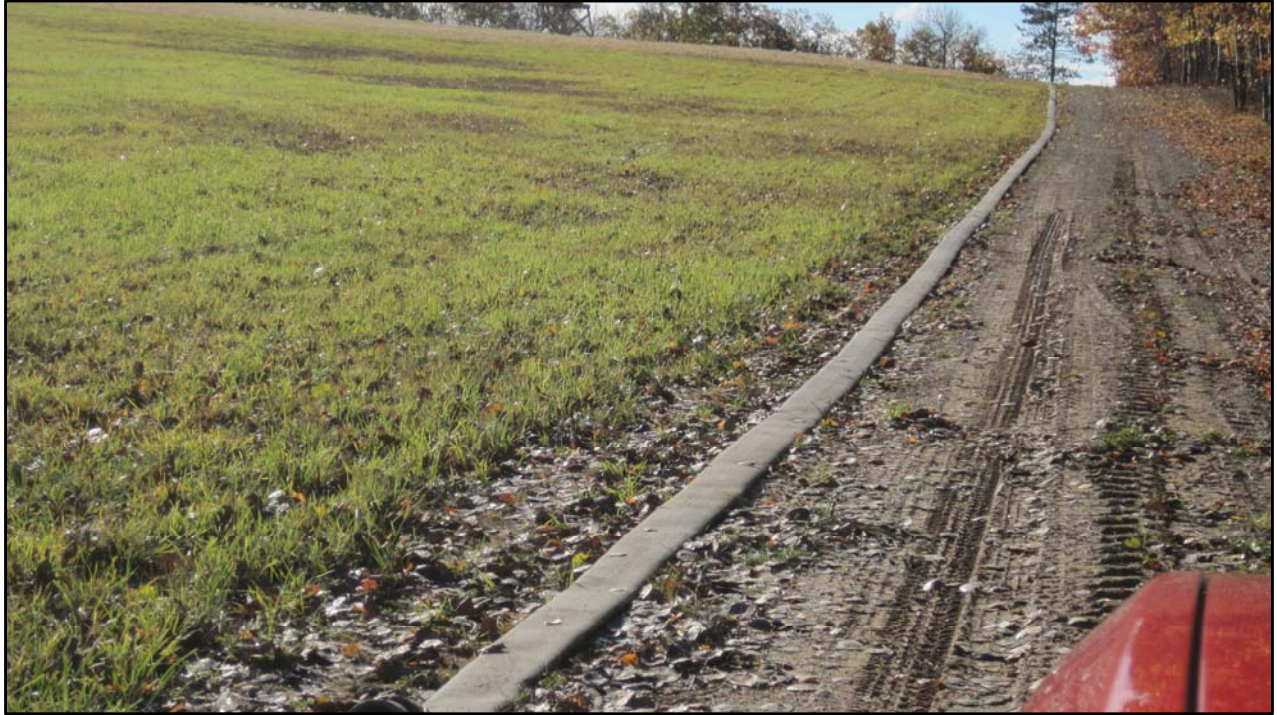
HOSE PROR TO PRESSURIZING
