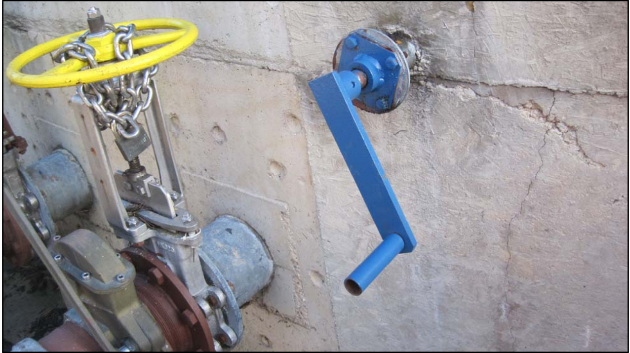
CRANK USED TO ROTATE PRESSURIZED AGITATER NOZZLE IN THE BOTTOM OF THE TANK
