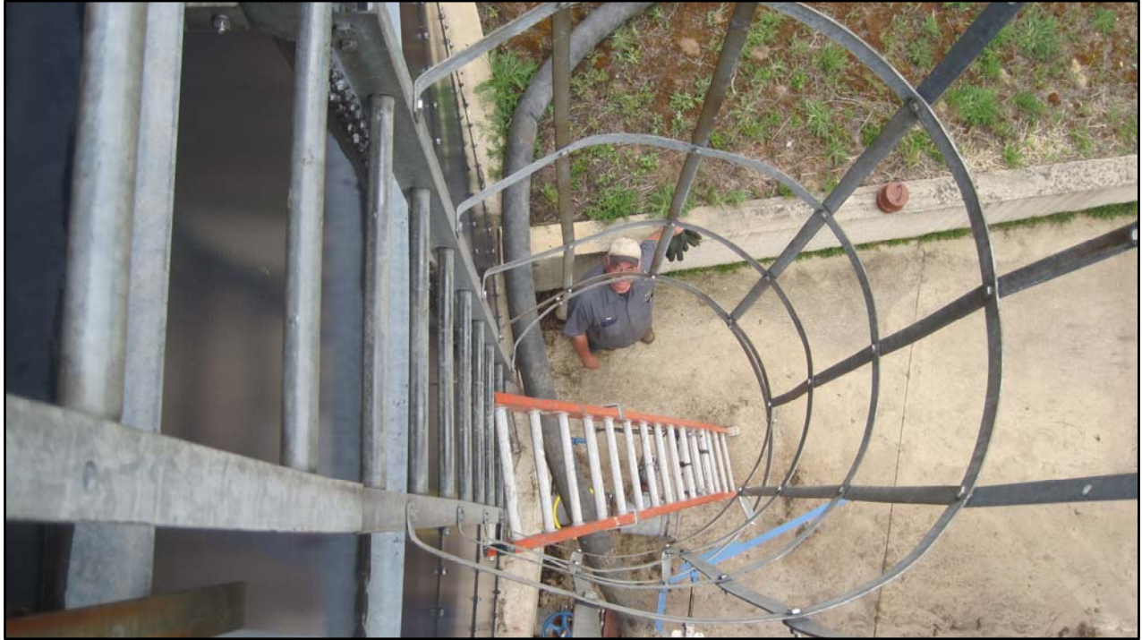
VIEW FROM THE TOP OF THE CATWALK
