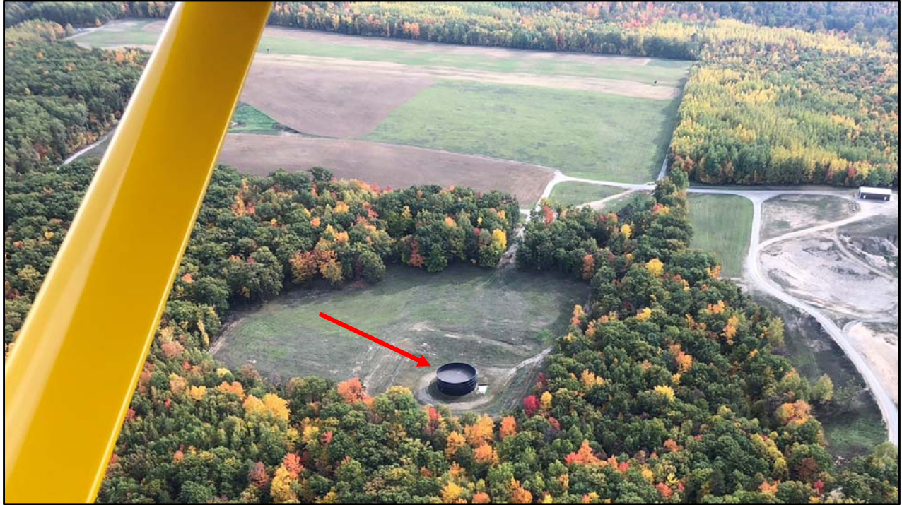
520,000-GALLON SLURRYSTORE – ABOUT \frac{3}{4} -FULL
